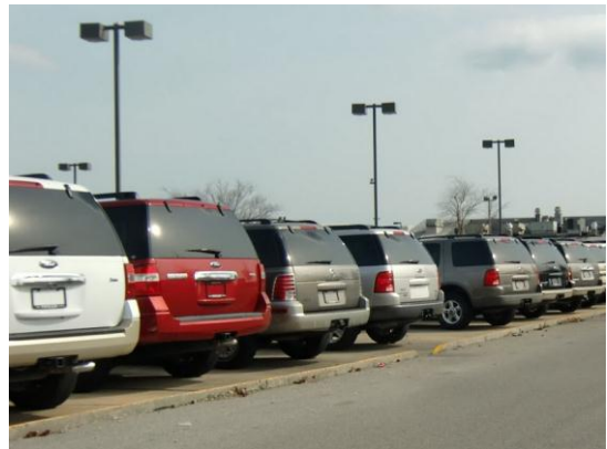
This is an example of good site lighting that uses "full cut-off" fixtures to minimize light spillage
